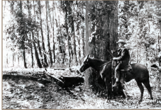
View along one side of New Madrid fault “fissure” near the banks of the St. Francis River in Clay County, Arkansas. © Courtesy of U.S.G.S.
