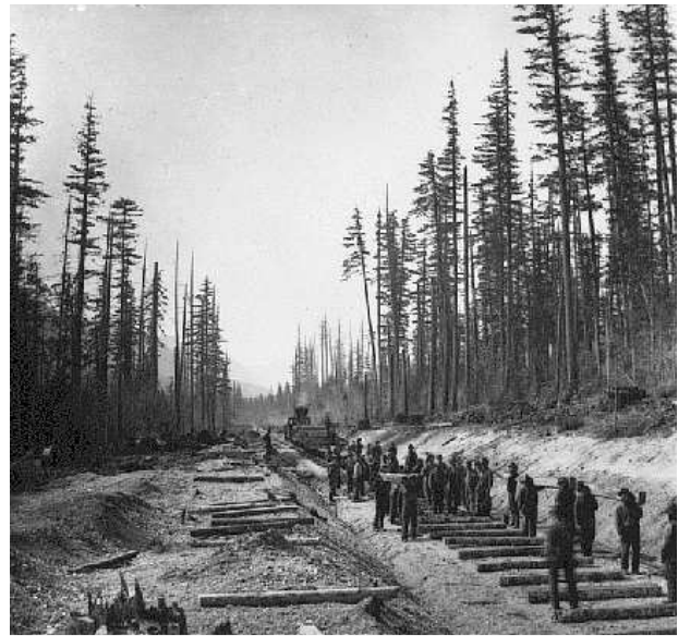
Workers laying the last section of track for the Canadian Pacific Railway
