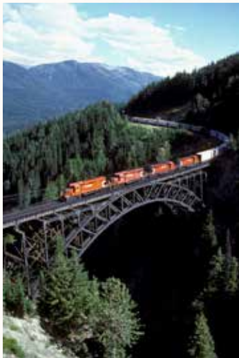
Stoney Creek Bridge at Rogers Pass
